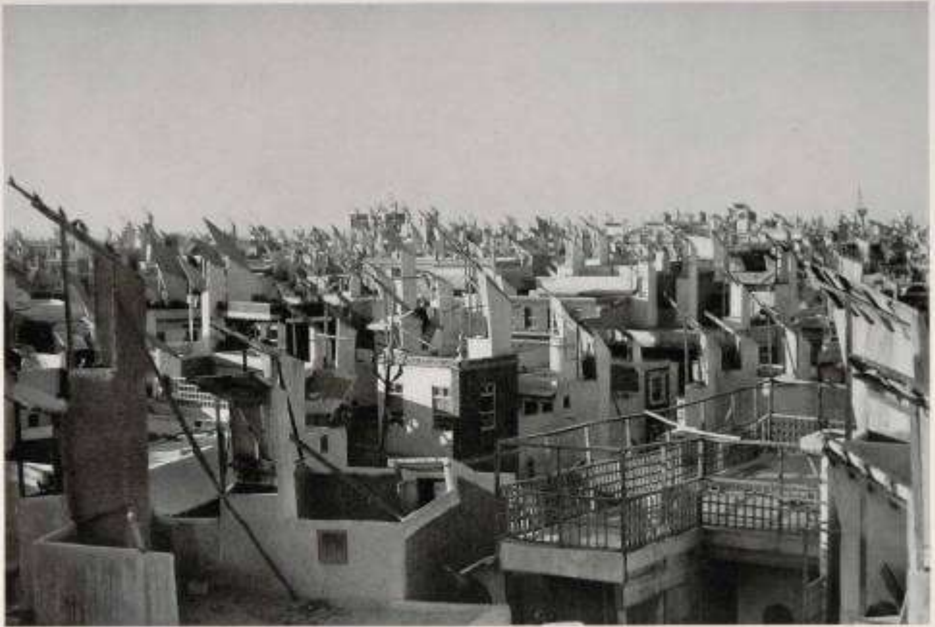
Rudowsky Architecture Without Architects
