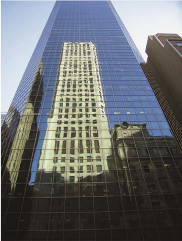
Fig. 2. Mirror facades darken the interior, making it necessary to switch on the lights during the day [21].
