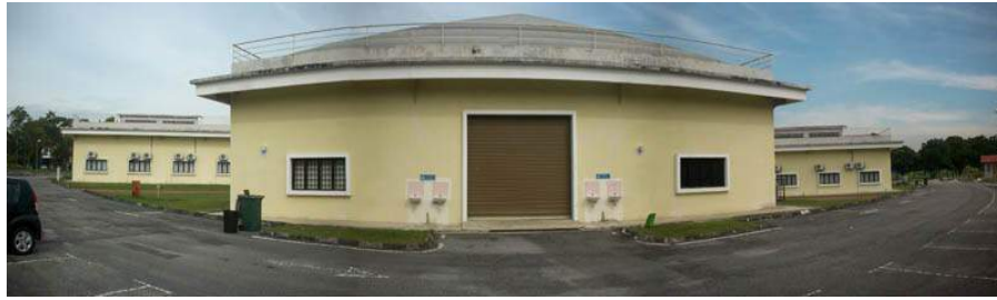
Figure 4.50 Studio 3 Industrial Design Building
